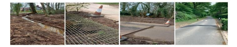
This enables the rainwater to flow into an existing open trench and away from the course beneath Lilyhurst Road. The excavation was then tarmacked twice, and the excess tarmac was used by Stave-Con to repair some of the potholes adjacent to the clubhouse and the north car park.
